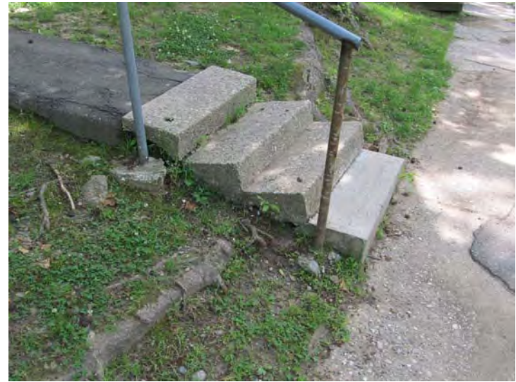
Concrete stairs providing access to unit entry walk have settled over time and require rebuilding
