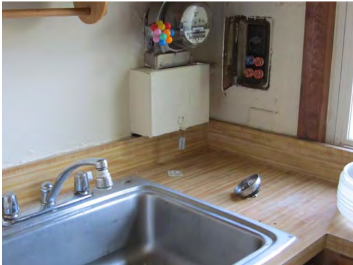
Location of fuse-equipped electrical load center and electric meter, adjacent to kitchen sink, are not compliant with current codes
