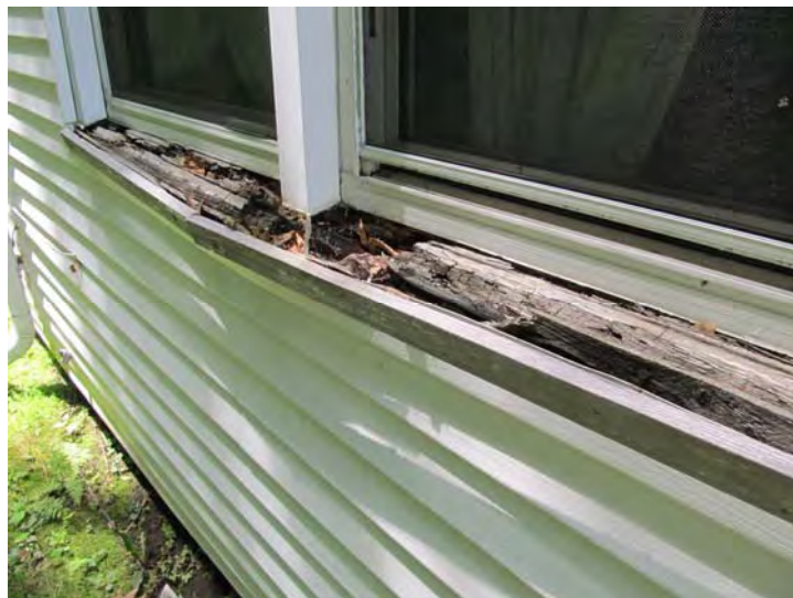
Original, water damaged, wood windowsills were clad with aluminum at some locations concurrent with installation of vinyl siding or window replacement work
