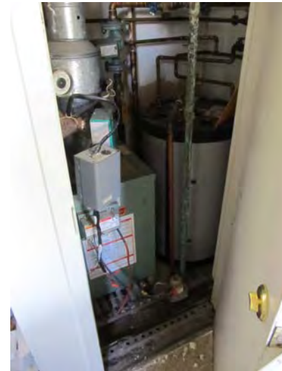
Typical natural gas-fired boiler and indirect-fired domestic hot water tank found at each unit
