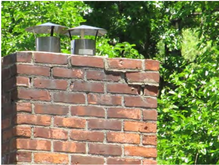
Brick chimneys exhibit mortar loss/ displacement at some locations
