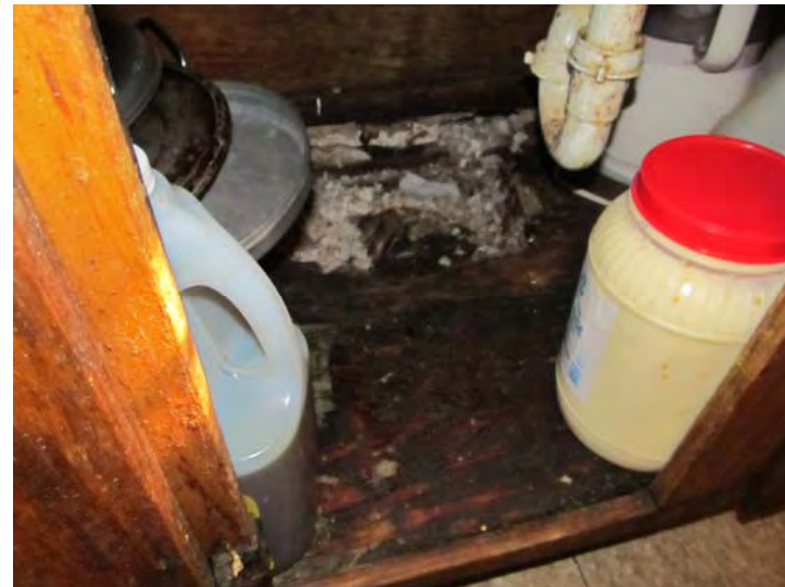
Damaged floor of base cabinet at kitchen sink
