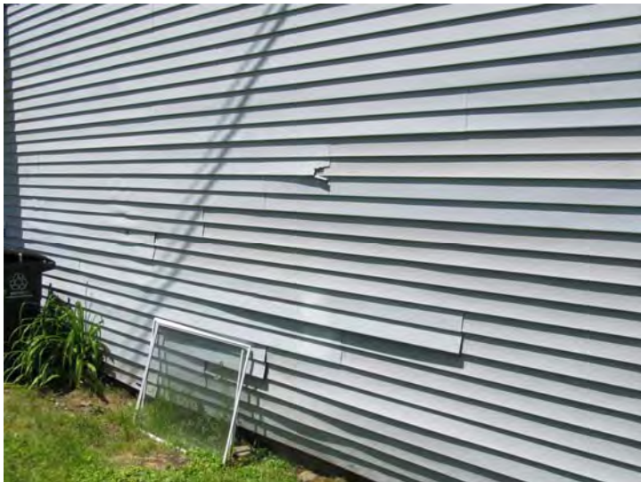
Vinyl siding exhibits age-related wear, impact damage, and loose seams at various locations
