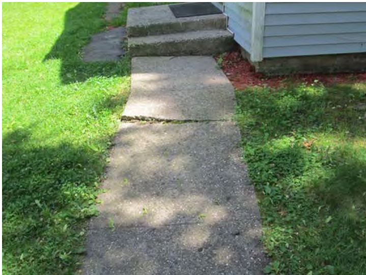
Need for sectional repair/replacement of walkways widespread throughout the development
