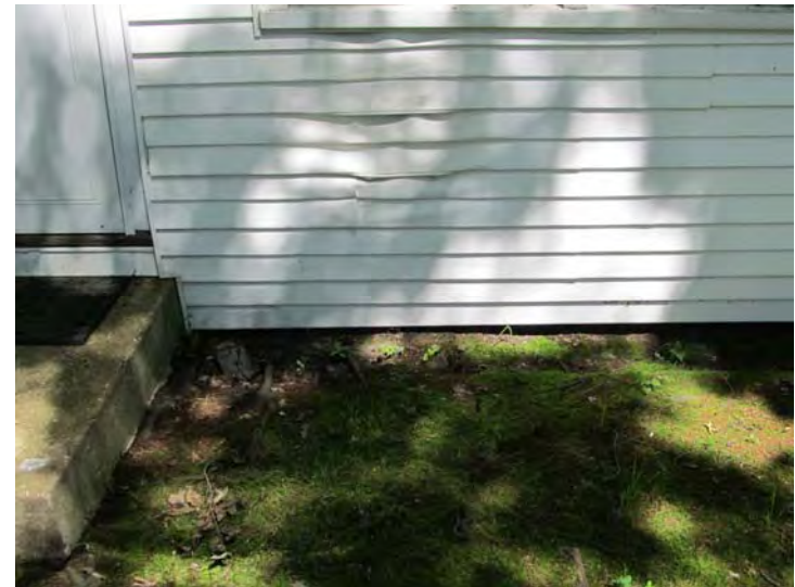
Heat damage noted on vinyl siding at various locations
