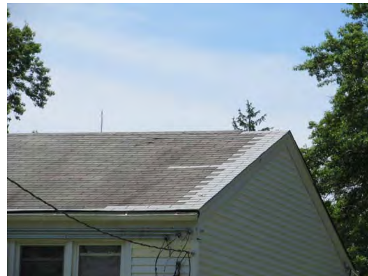
Three-tab shingles on roof surfaces vary in condition with some evidence of past repair efforts evident
